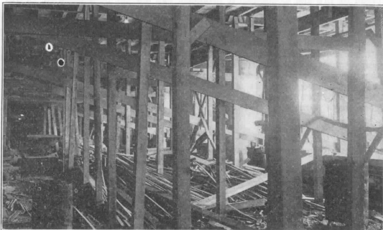
Reinforced concrete building with wooden shoring in place; also, large quantity of combustible refuse.
