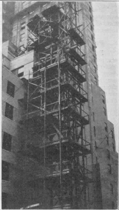
Combustible scaffolding 23 stories high. Near view of lower portion of picture on the left.
