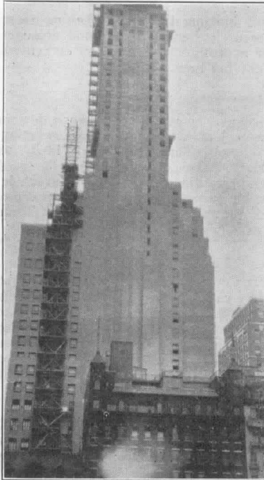
Combustible scaffolding for lower 23 floors; steel scaffolding and flame-proofed planking on upper floors.
