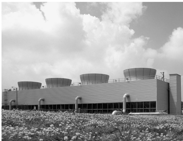
FIGURE B.1(d) Typical Induced-Draft Counterflow Water-Cooling Tower.
