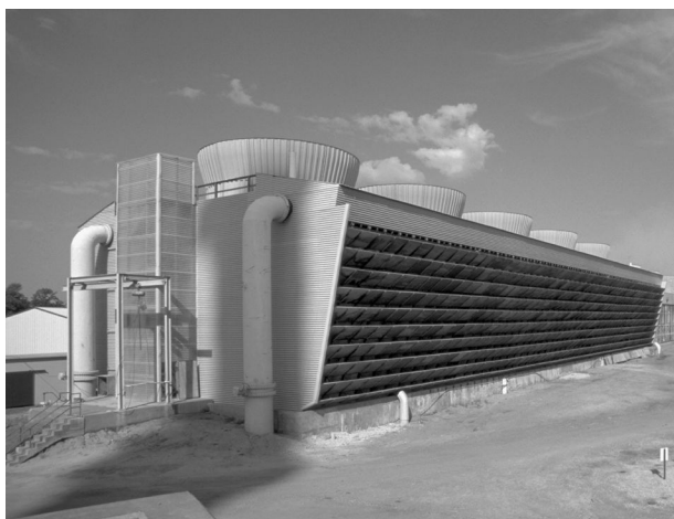
FIGURE B.1(e) Typical Induced-Draft Crossflow Water-Cooling Tower.
