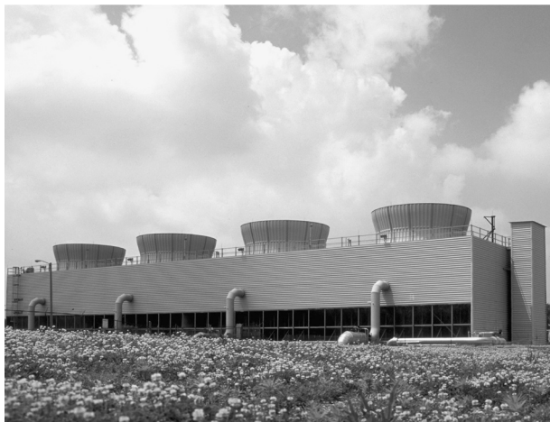
FIGURE B.1(d) Typical Induced-Draft Counterflow Water-Cooling Tower.
