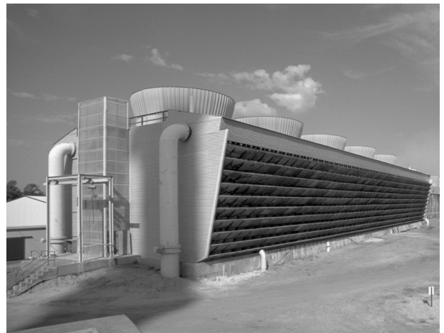
FIGURE B.1(e) Typical Induced-Draft Crossflow Water-Cooling Tower.
