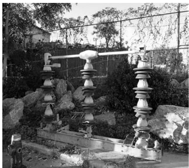
FIGURE A.8.3.6.2 138 kV Substation Disconnect Switch. (Courtesy of ConEdison.)
