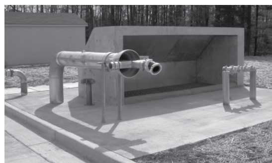
FIGURE B.7.3.1 Outdoor Drafting Pit. (Courtesy of Woodman Road Fire Training Center, Henrico County, VA)
