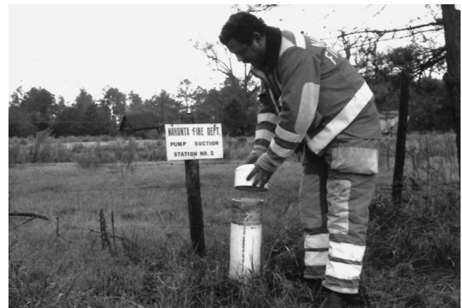
Figure B-5.6(a) Dry hydrant innovation that has eliminated top 90-degree or 45-degree elbow. (Courtesy of Nahunta Volunteer Fire Department, NC)
