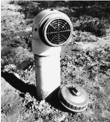
Figure B-5.1 Dry hydrant.
