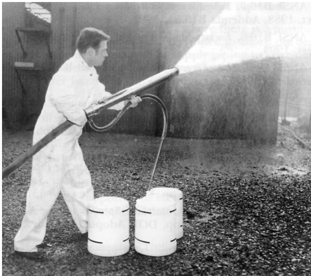
FIGURE A.3.3.24.3(b) Air Foam Hose Nozzle with Built-in Eductor.
